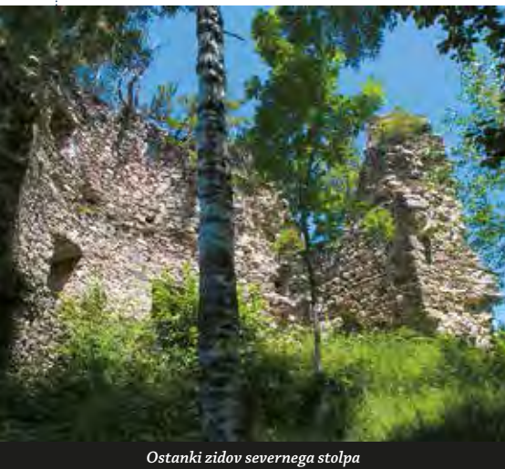
Ostanki zidov severnega stolpa
